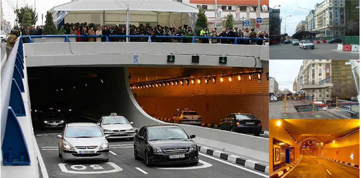
The subterranean roadway is composed of two independent twin tunnels which have two lanes in each direction, connected by emergency exits every 100m.
